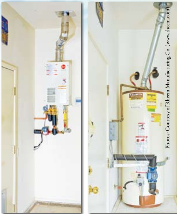
These photos illustrate the difference in space requirements for a tank-type water heater versus a tankless.
